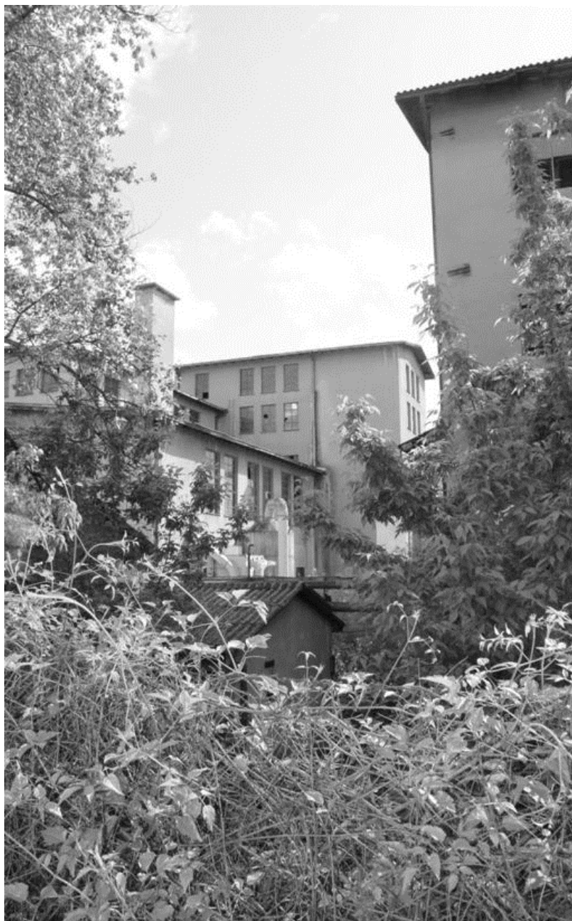
Figure 03. Kuprum Factory – Author photography, 2021.
